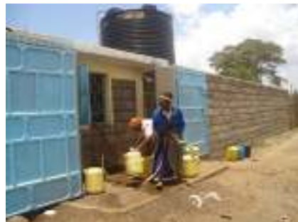
The new wall and security gates for the borehole
